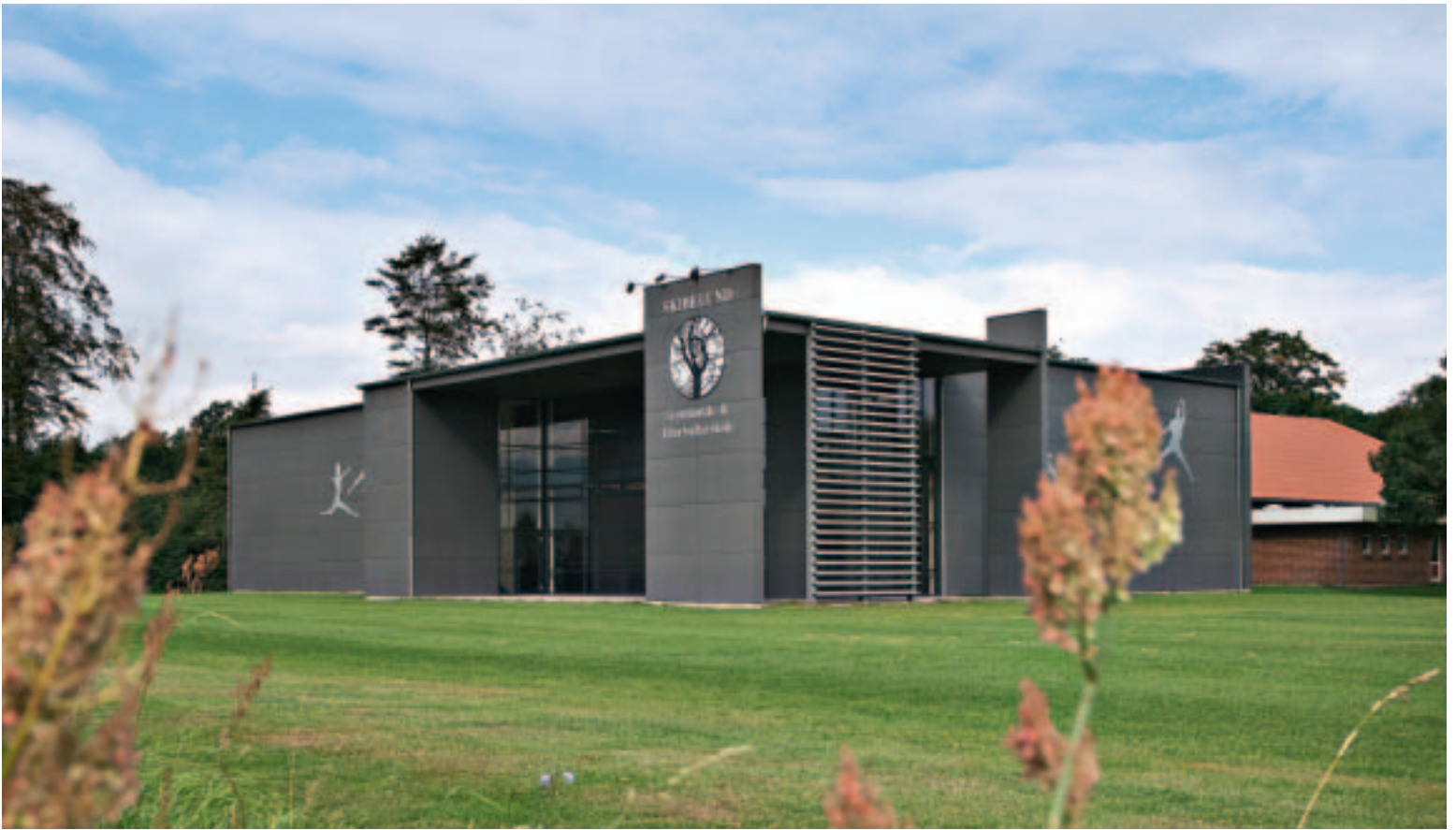
Extension of Skibelund School for Gymnastics and Athletics, Vejen, Denmark A New Face for the School
